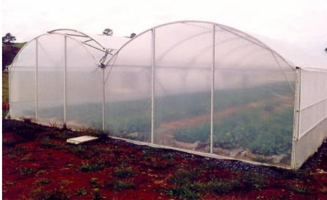
This provides efficiencies in both performance and cost. The roof vents are operated automatic electric motor gearboxes as a standard feature. A selection of computer controllers is available for accurate monitoring and control. The 7500 FI vented arch model (pictured above and left) also includes the Redpath Eziwinder roll up sidewall ventilation system for the full length of both sidewalls as standard. These are
