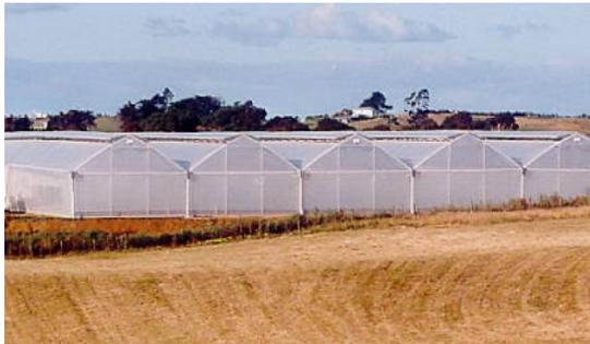
Redpath's Super-Twin design has been developed to meet the many needs of the modern grower. This structure's cosecant curved rafter design has been developed by Redpath in line with the latest overseas technology and has many fundamental advantages over traditional straight rafter designs.
